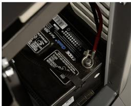
Clean and tighten battery terminals.
